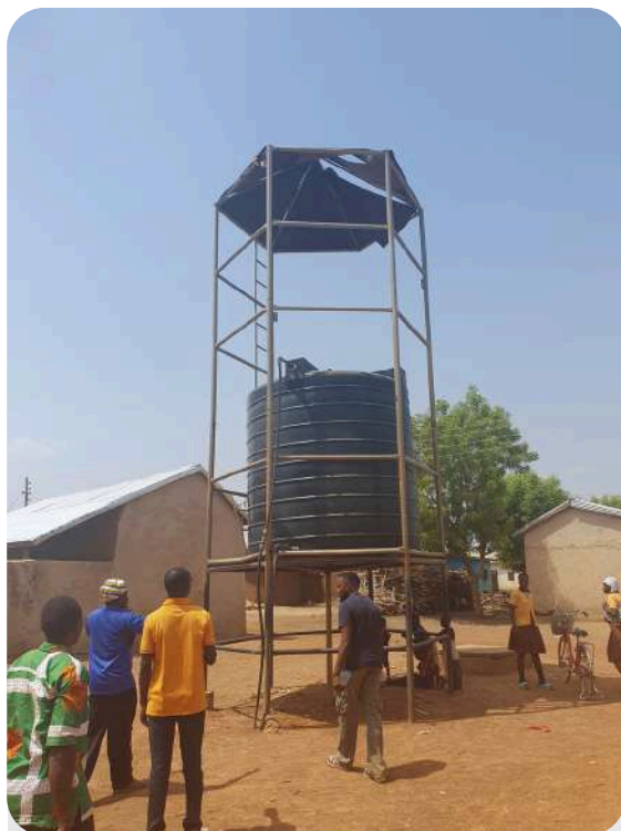
An elevated water tank in a rural Ghanaian community, surrounded by locals, supporting improved water access under the EnWASH program.
